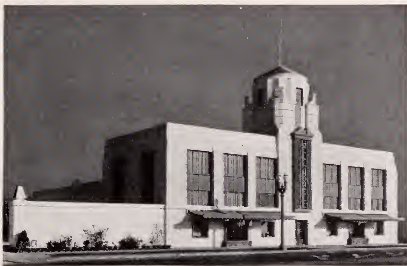
• To extend and increase Bell & Howell service to the industry, our new Hollywood home at 710-724 North La Brea Avenue is dedicated. With its complete engineering, research, and service facilities, it will supplement and assist the famous Bell & Howell research and engineering department at Chicago.
